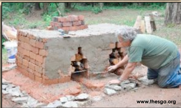
Top: Artist reconstruction of a small-scale brickmaking operation including a brick clamp. Bottom: Mock brick clamp with three benches and two flues on a clay floor.
